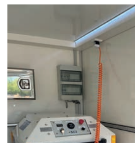
Image: Trailer with fixing system, socket strip and LED light rail
