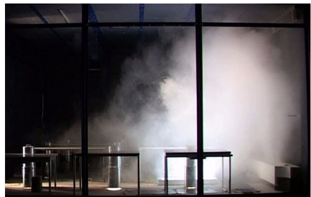
Example of room air flow: VFC-N with special fan insert for mixed air/displacement air
